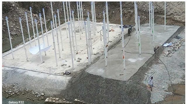
Concreting of foundation of block in stilling basin.
