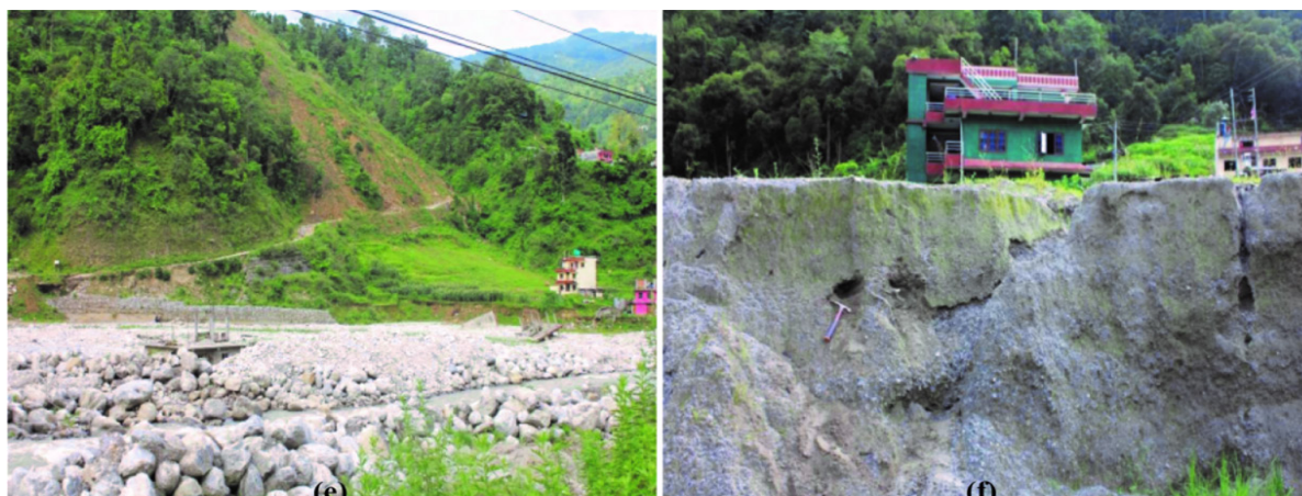
Fig. 9: Damaged bridge, houses, sand bar observed between Gyalthum and Danuwar gaun. (a) landslide opposite Gyalthum with baily bridge, (b) Melamchi khola bar SW of Gylthum, (c) Collapsed building at left bank of Melamchi river at Thulokhet, (d) Sand bar on top of boulder, (e) Destroyed building of Danuwar Gaun (f) Fine particles deposietd on 3m high bar near damaged bridge abutment.
