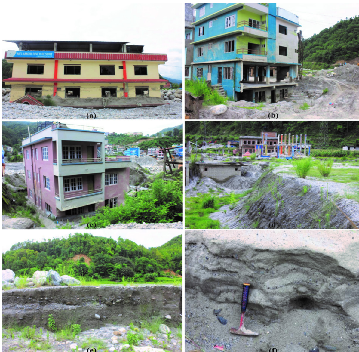
Fig. 10: Buried houses, flood mark, debris flow deposits, sand bar observed below Danuwar gaun and Dolalghat. (a) Buried Melamchi river resort, (b) High flood mark on green blue buildings, (c) Houses buried on two floors on Melamchi bazaar, (d) Debris flow deposits at the transverse from Melamchi to Dolalghat area, (e) Deposits of Crudely stratified sand bed at Bahunepati, (f) 30 cm thick sand bar near Sipaghat at Eklebesi, Magitar
